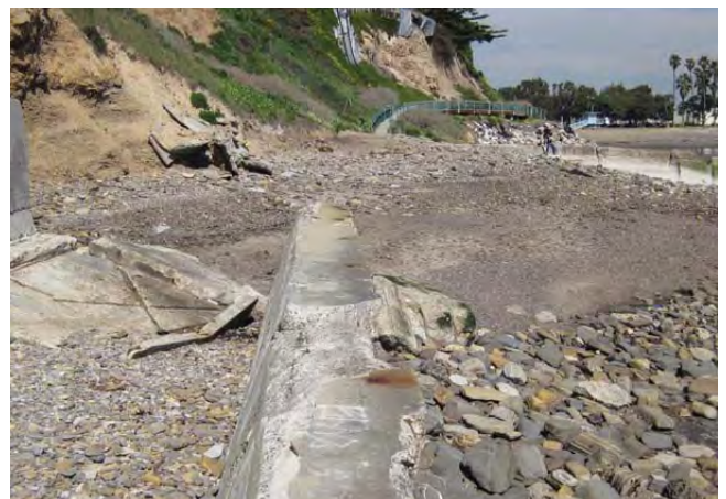
Figure 3. Looking back towards park from concrete bunker.
